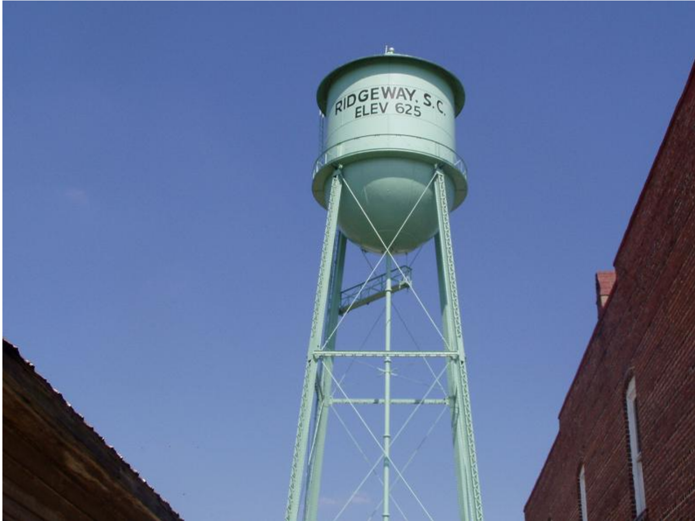
Built in the 1920s, Ridgeway's "Tin Man"-style water tower is visible from the shops of the downtown.
